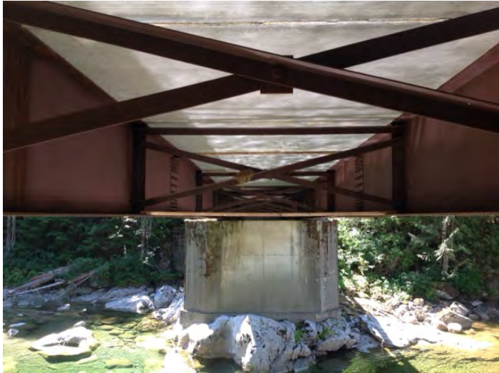
main span superstructure
