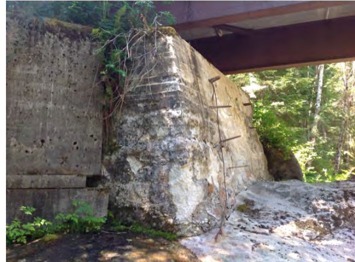
Right Bank Abutment when facing downstream
