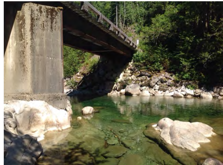
Left Bank Abutment when facing downstream
