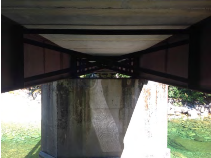
jump span superstructure
