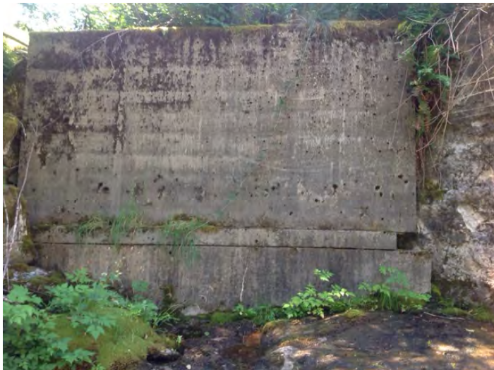
right downstream wing wall
